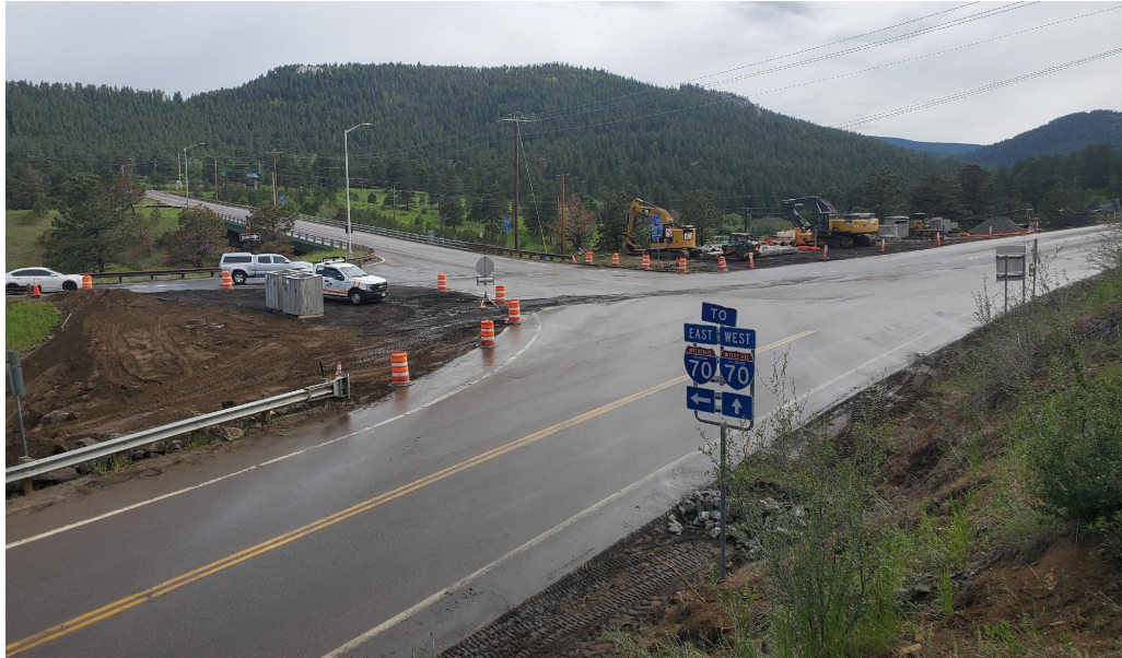
(Pictured Above: Current stage of roundabout construction at US 40 and CR 65)
